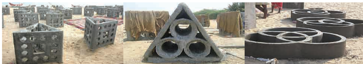
Fig.2. Three types of modules, 70 each form a cluster, occupying 1000 m 2 area, with about 500 m 3 volume and provide about 3000 m 2 surface area for attachment of marine organisms
